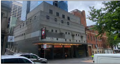
Figure 23: Existing conditions to Lonsdale Street
